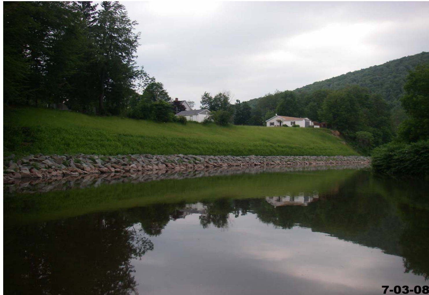
Village of Walton - Terrace Avenue Streambank Restoration - 2007
