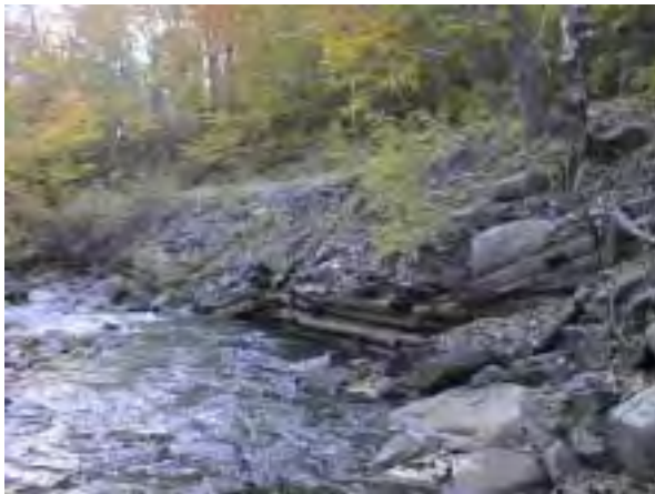
Photo 6. Example of Nonfunctioning Condition
