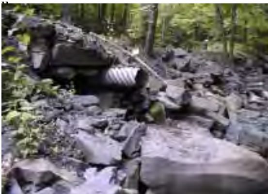
Photo 4. Culvert in lower rip-rap section, right bank, MU1.
