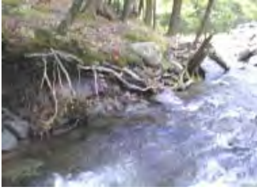
Photo 5. Minor bank erosion, across from lower rip-rap section, MU1.
