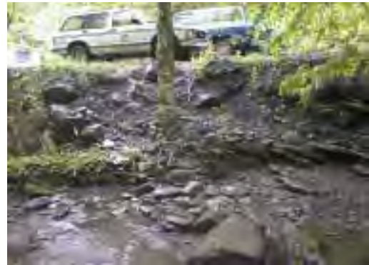
Photo 6. Minor bank erosion, NYSDEC turnout, MU1.
