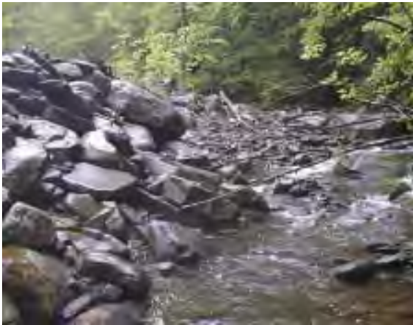
Photo 2. Looking upstream at un-vegetated boulder rip-rap.
