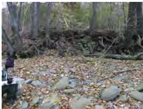
Photo 8. Eroding bank at forested floodplain on left bank, just above lower rip-rap section at the bottom of MU7, monitoring cross-section 17.
