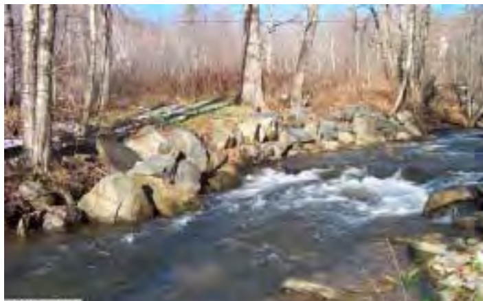
Photo 7. Looking upstream at stacked rock wall revetment on the right bank of MU 7.
