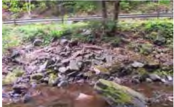
Photo 6. Right bank dumped rock fill, along Broadstreet Hollow Road embankment near the top of MU10. Stream flow is from right to left.
