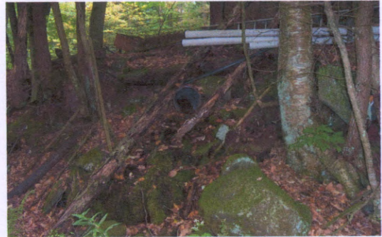
Photo 9. Corrugated culvert in left bank landfill/dumping site. Stream is behind the viewer, flow from left to right.
