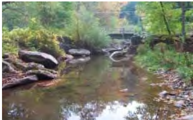
Photo 4. Looking upstream toward County bridge 2-22457-0. Willows just downstream from the bridge (at the left) may help prevent further bank and stream bed erosion, while allowing the passage of water through them during floods.
