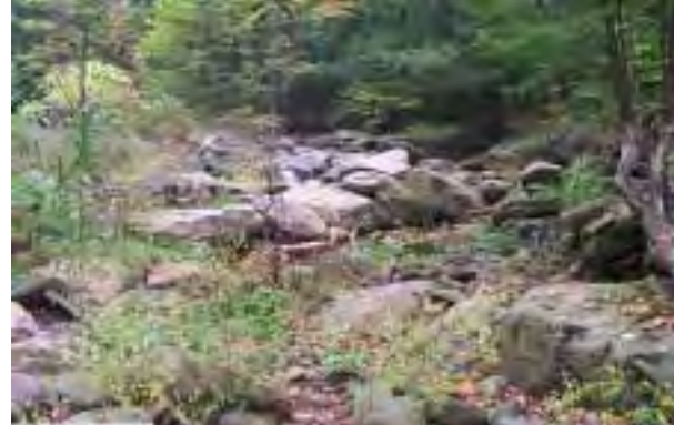
Photo 4. Looking upstream into the top of the main side channel at the top of MU13, the 108 Broadstreet Hollow Road hillside is to the left outside the frame, boulder berm in the center background.
