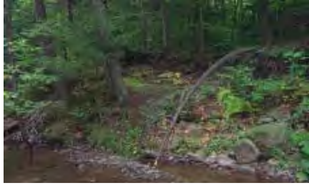
Photo 5. Left bank, upstream from area in Photo 4. Note trees leaning toward the stream, a long crack in the hillside behind them, parallel to the stream, demonstrating the downslope streamward motion of large sections of the hillside, held together by tree roots. Stream flow is from left to right.
