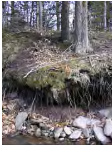
Photo 7. Close-up of eroding left bank, showing deep undercut forming a "shelf" held together by dense tree roots. The shelf is up to five feet deep, straight back into the bank. Note reddish clay exposure above the stream cobbles. Stream flow is from left to right.
