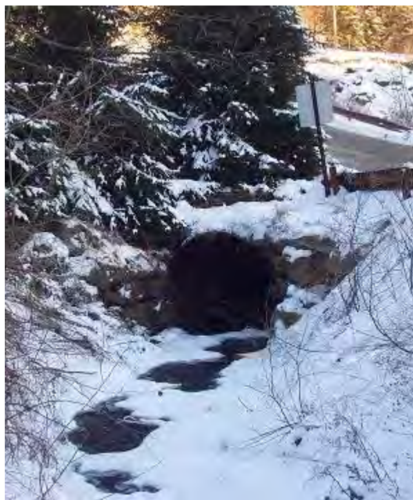
Photo 14. Tributary through culvert under Meyers Rd.
