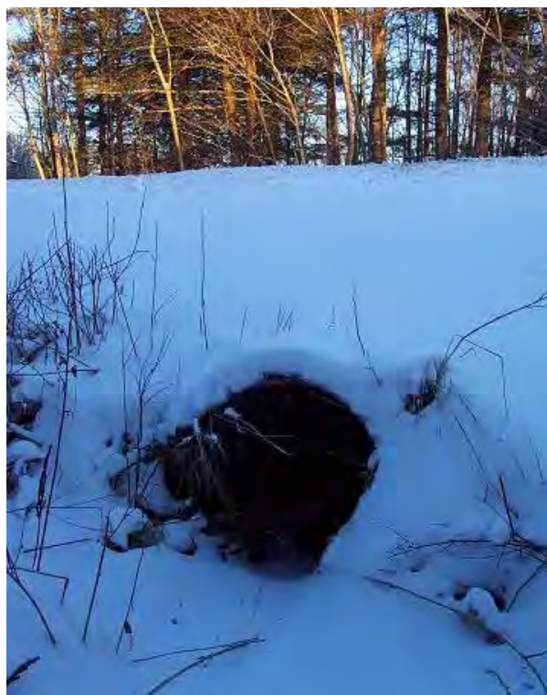
Photo 13. Tributary through culvert, Mutton Hill Rd.
