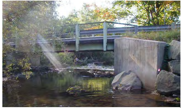
Photo 7. Looking downstream at right span of Davis Lane Bridge.
