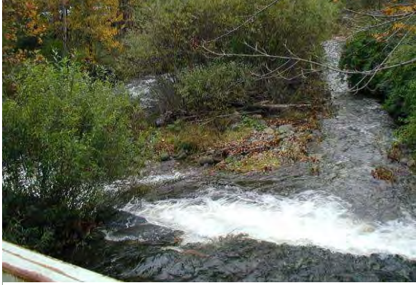
Photo 10. Looking downstream from top of Davis Lane Bridge at split channel below grade control at high flow. Right channel dry in 2001 at low flow. Center bar with cobbles and willow can be seen.
