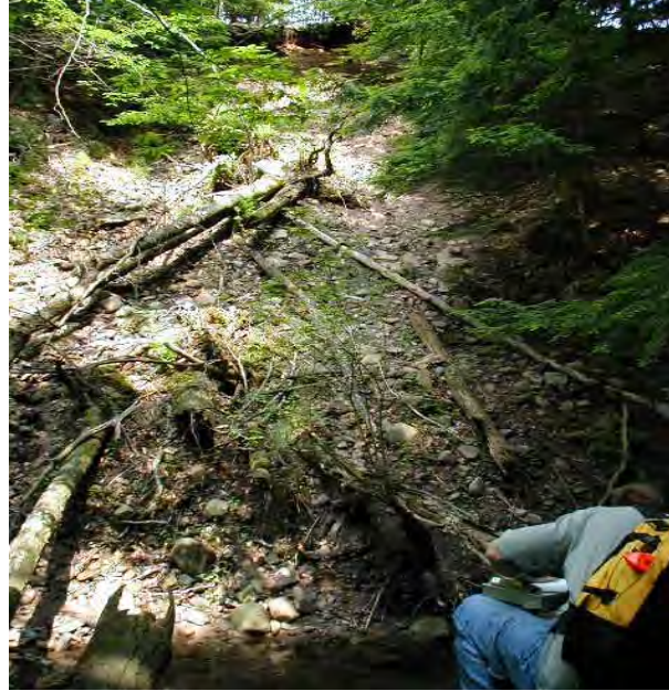
Photo 16. Shows very steep eroding right bank along the upper reaches of Pepacton Hollow along Camp Road.
