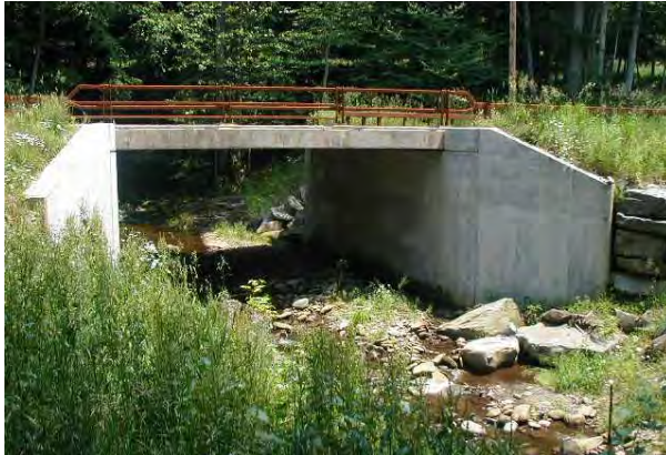
Photo 6. Looking upstream at County box culvert Pepacton Hollow Rd.
