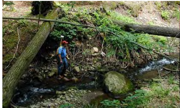
Photo 17. Eroding right bank and fallen trees, incised section, along Camp Road.
