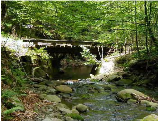
Photo 5. View looking downstream toward Slater Bridge and Camp Road.
