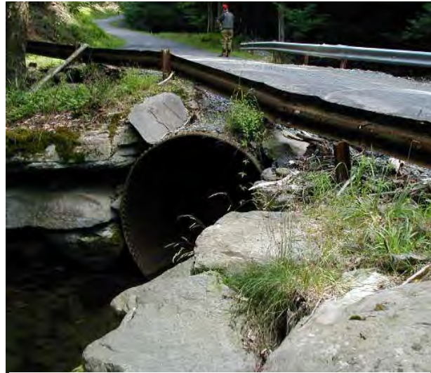
Photo 7. Culvert crossing under Pepacton Hollow Road.
