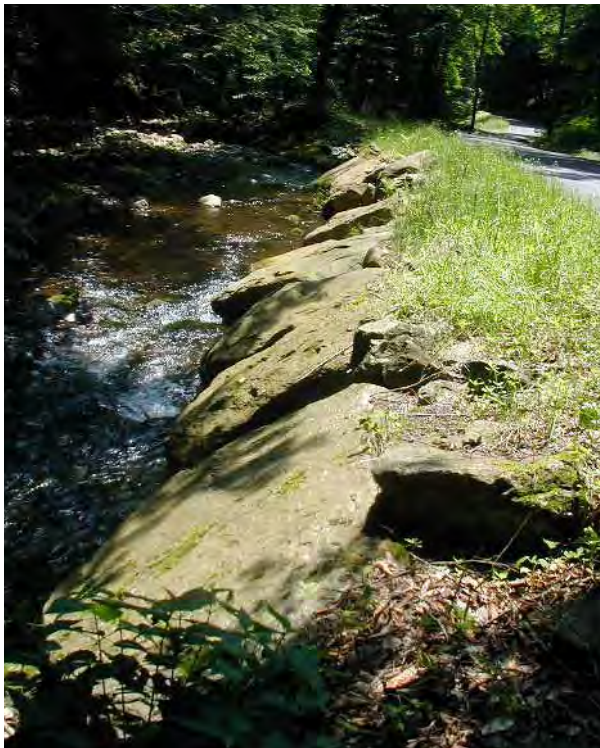
Photo 9. View looking downstream at riprap on right bank.
