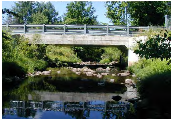
Photo 3. DEP bridge over Red Brook.
