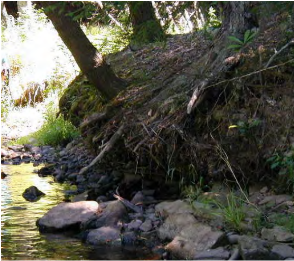
Photo 10. View looking at erosion and undercut trees on right bank.
