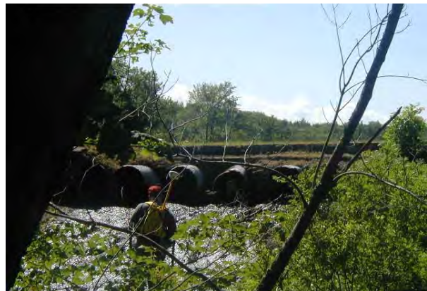
Photo 2. Beaver Dam Pond outfall. Six Culverts, looking upstream.
