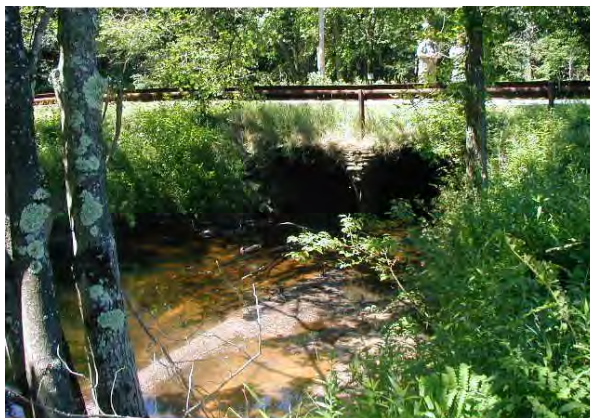
Photo 5. Looking upstream at twin culvert Beaver Dam Road crossing.
