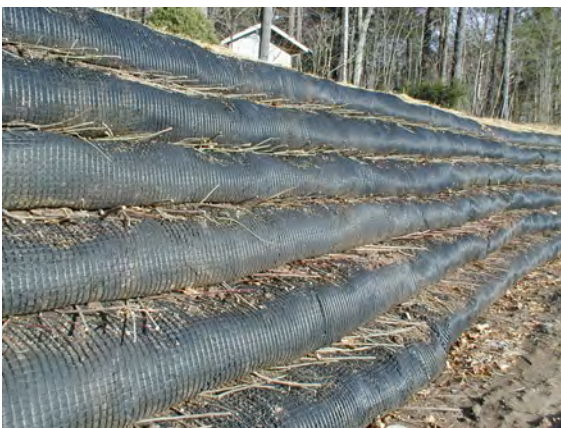
Figure 20. VRSS - geotextile encapsulated soil lifts with layered willow whips (12.05.03)
