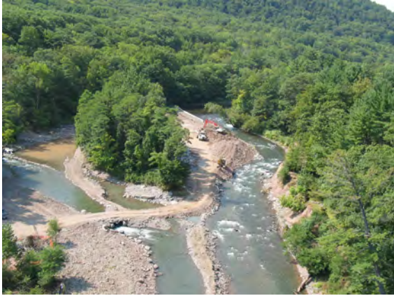
Figure 9. Aerial view of project construction (9.11.03)
