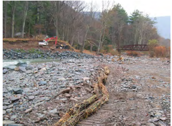
Figure 17. Willow fascine placement along cobble bar (11.19.03)
