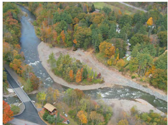
Figure 15. Aerial view of project reach after channel restoration (10.16.03)
