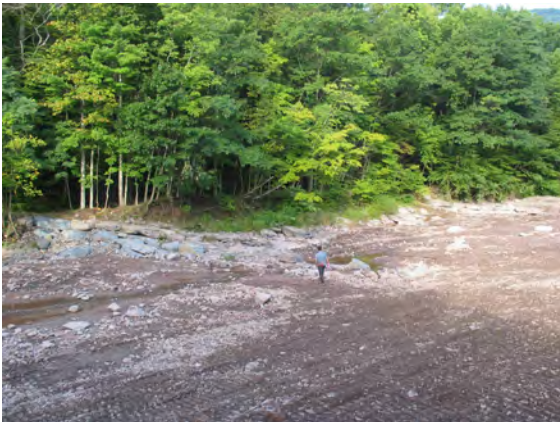
Figure 8. Completed south channel with upstream weir (9.09.03)
