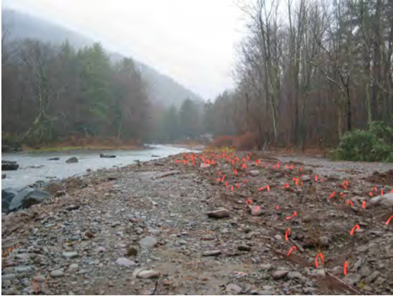
Figure 16. Tree plantings along the new channel margin (11.19.03)
