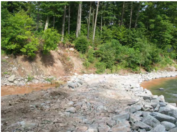
Figure 11. Constructing downstream channel block (9.18.03)
