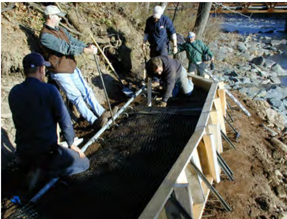
Figure 18. Constructing VRSS with batter boards (11.11.03).
