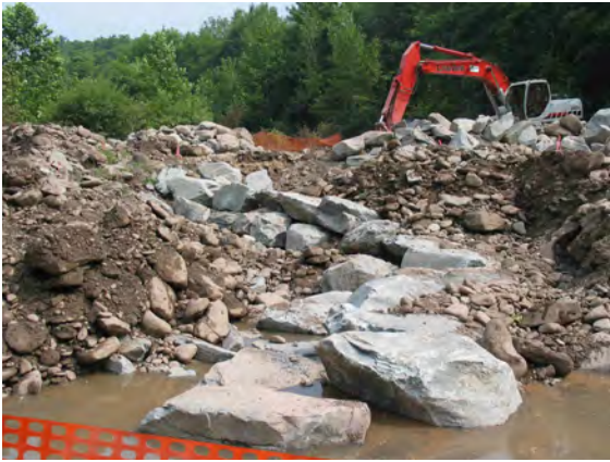
Figure 6. Constructing rock vane and weir below Woodland Valley confluence (8.20.03)
