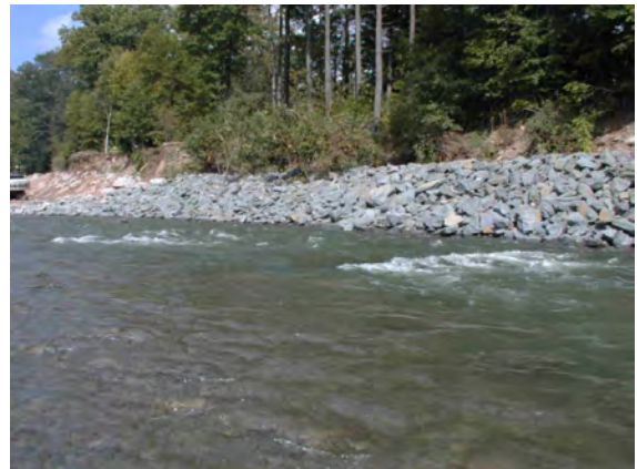
Figure 12. Rip rap revetment along failing bank (9.24.03)
