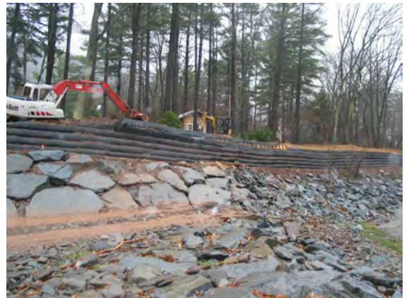
Figure 19. VRSS on top of rip rap at downstream channel block (11.24.03)
