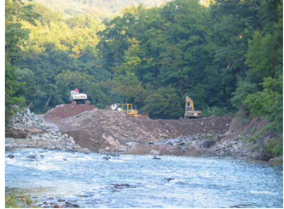
Figure 10. Filling in cutoff channel (9.17.03)
