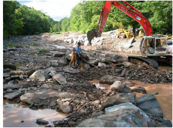
Figure 7. Excavating new channel and constructing rock vane (9.x.03)
