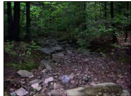
Flood chute at Station 80700
