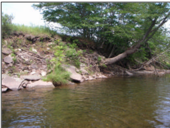
Erosion at Stations 50676 - 50471
