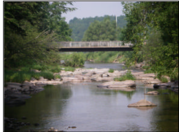
Bridge at Station 40131
