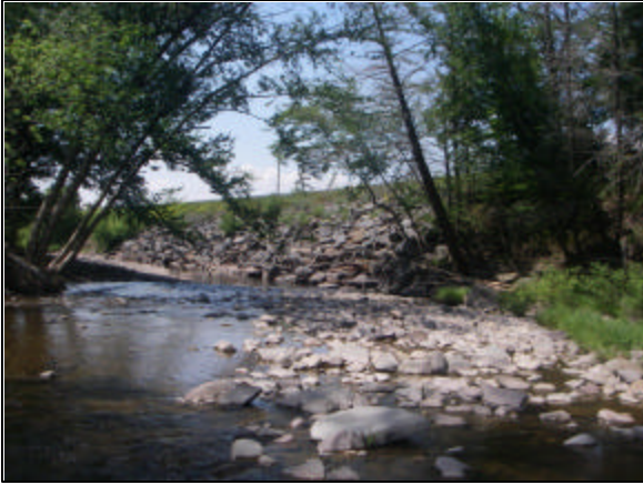
Rip-rap at Stations 41789 - 41587
