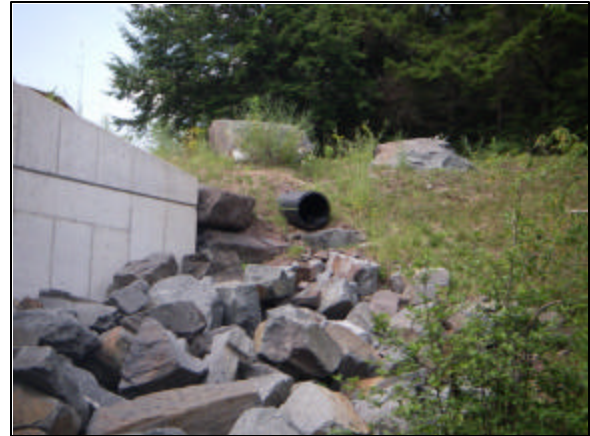
Piped outfall at Station 51070
