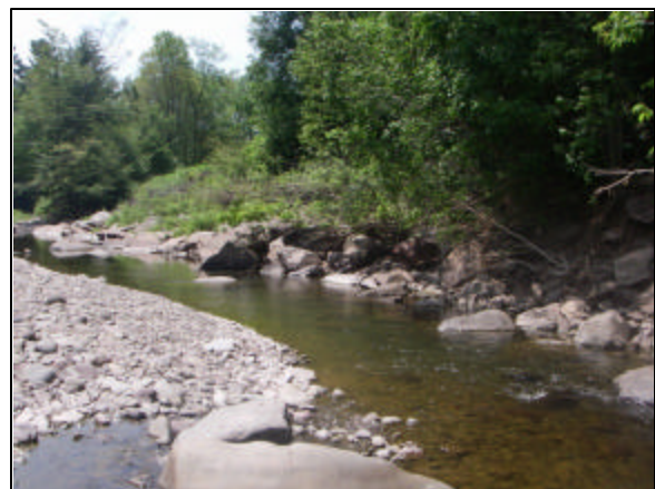
Rip-rap at Stations 42923 - 42713
