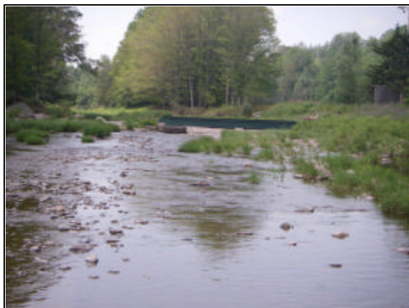
Bridge at Station 44190
