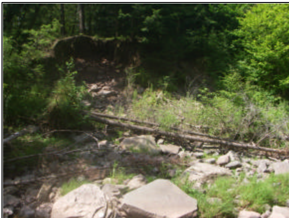
Mass failure at Stations 48400 - 48269
