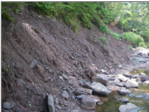
Mass failure & clay exposure at Stations 42407 - 42263
