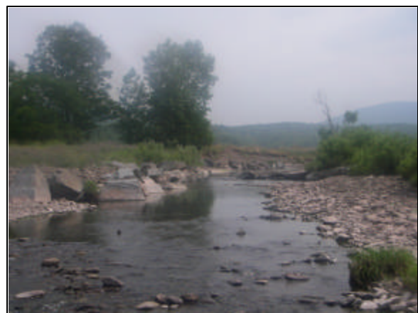
Cross vane at Station 38306 photo orientation – looking upstream
