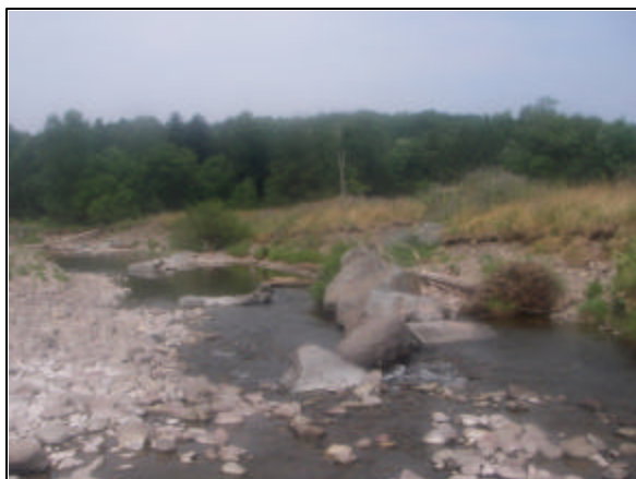
Erosion at Stations 38716 – 38401
