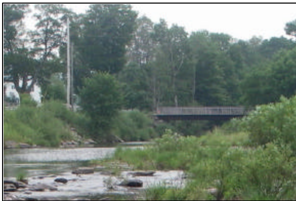
Bridge at Station 40130 photo orientation – looking upstream
