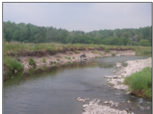
Erosion at Stations 39192 - 38901
