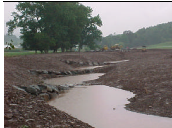
Rock vane construction - Summer 2000
