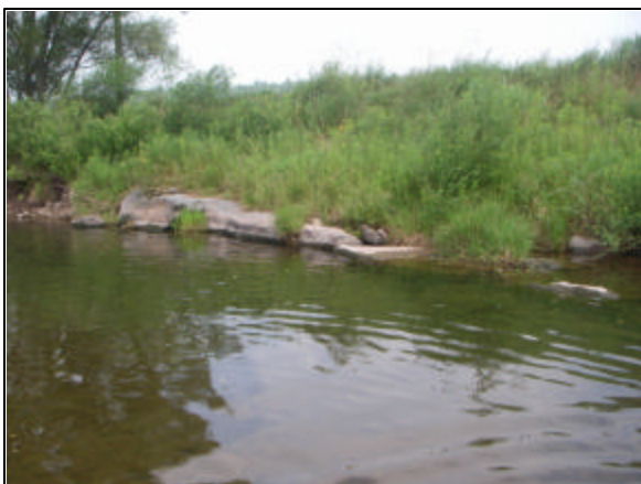
Rock vane at Station 39922
