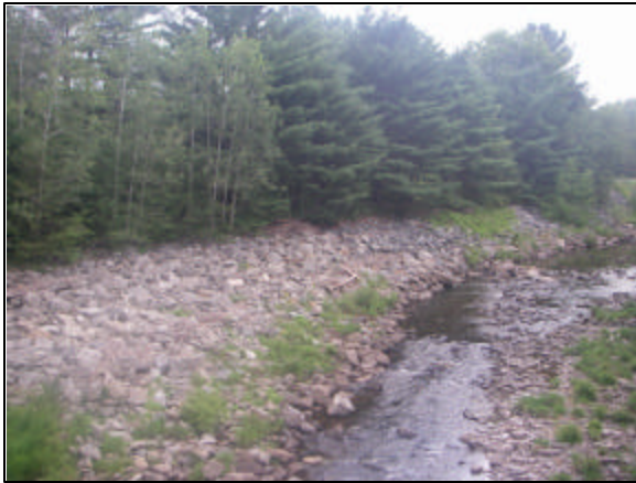
Rip-rap at Stations 27224 – 26386 photo orientation – looking upstream
