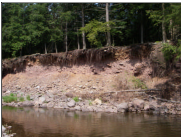
Mass failure at Stations 34559 - 34461
