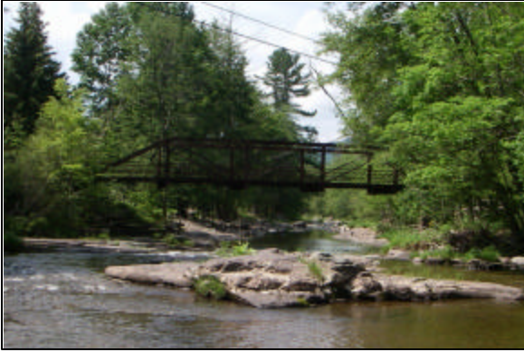
Bridge at Station 28817
