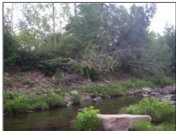
Erosion at Stations 28151 – 27800 photo orientation – looking upstream
