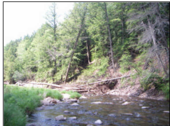
Mass failure at Stations 29657 - 29235
