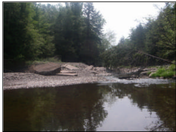
Concrete abutment remains at Station 34619
