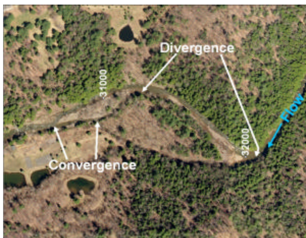
Split channel between Stations 32020 – 30665 Flood chute between Stations 31276 – 30900
