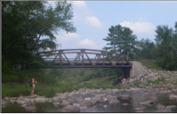
Route 296 Bridge at Station 26386
