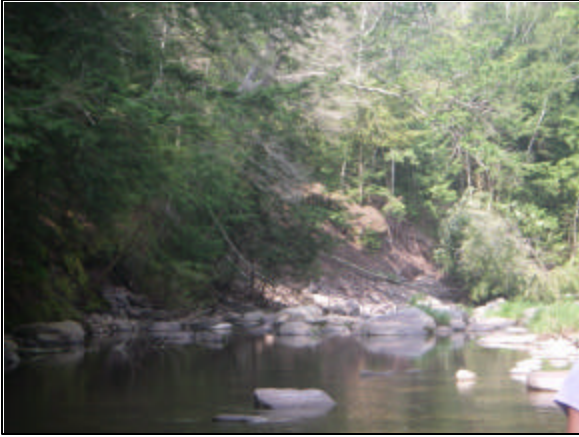
Mass failure at Stations 21427 - 21251
