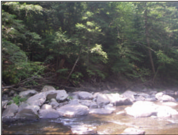
Erosion at Stations 16572 - 16332
