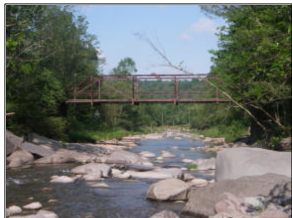
Mill Hollow Road Bridge at Station 11254
