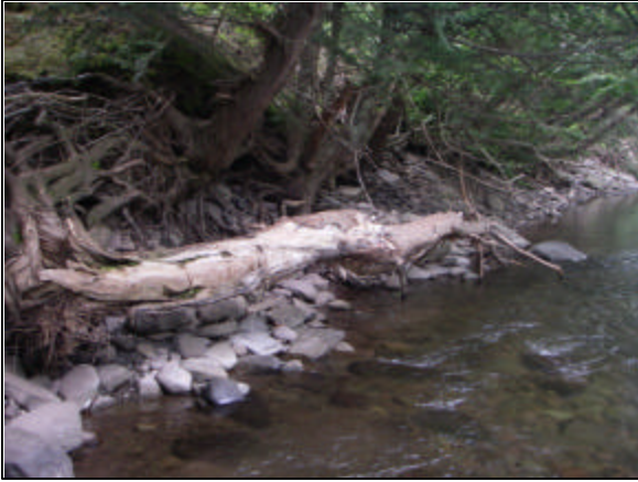
Woody debris at Station 14281 Erosion at Stations 14656 - 14093
