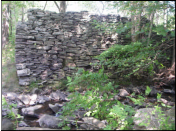
Rock wall and Roaring Brook at Station 11312
