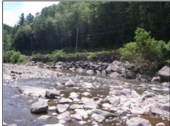
Revetment at Station 3540-3104
