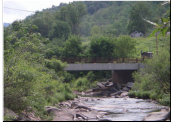
Mill Hollow Road Bridge at Station 6699
