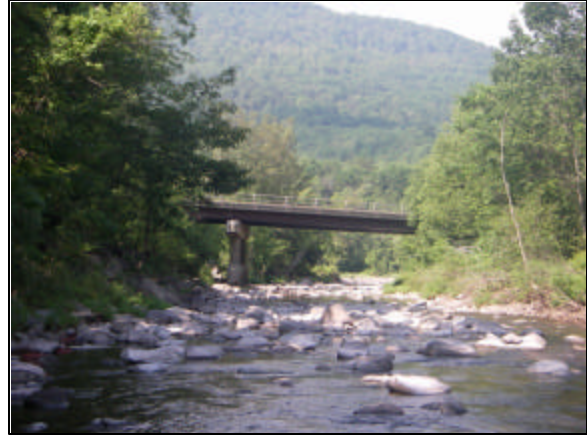
County Route 23A bridge at Station 300
