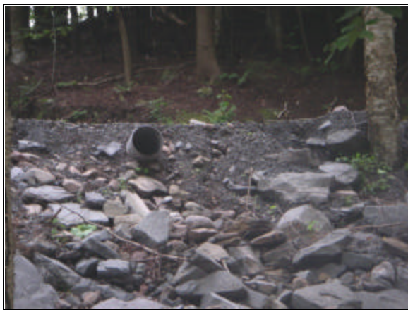
Piped outfall at Station 6260
