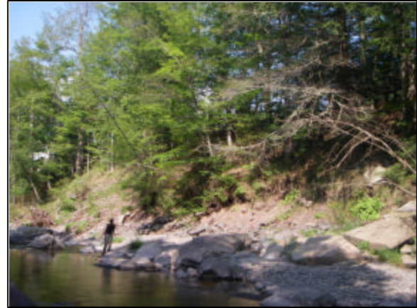
Bank erosion, BEMS #06EK2422 Stations 1470 - 1084
