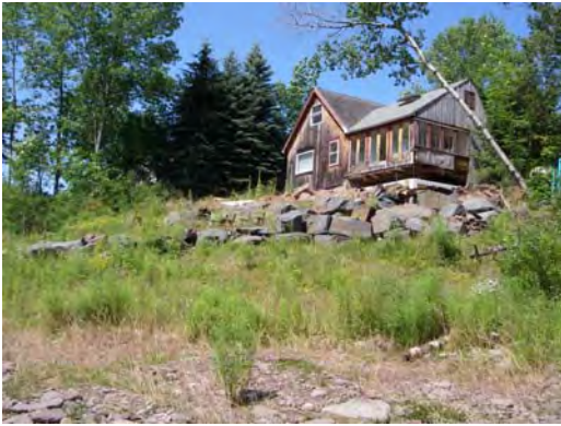
Streamside development and limited riparian vegetation leads to compromised streambanks. This bank has been reinforced with riprap.
