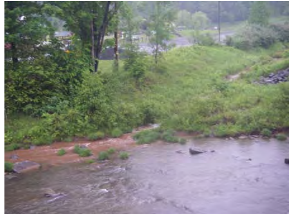
Turbid discharge from a road ditch as it enters the clear Schoharie Creek
