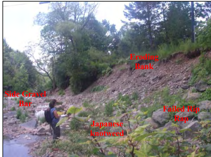
GCSWCD personnel assess a stretch of Schoharie Creek that includes many stream features examples.
