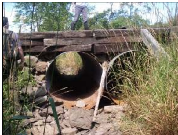
Bridge and Culverts at Station 46395
