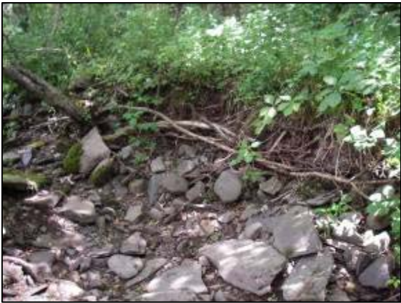
Eroding bank, Stations 48259 -48181
