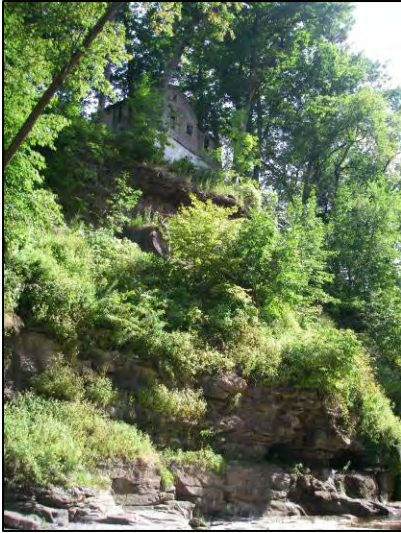
Waterfall House at Station 1100
