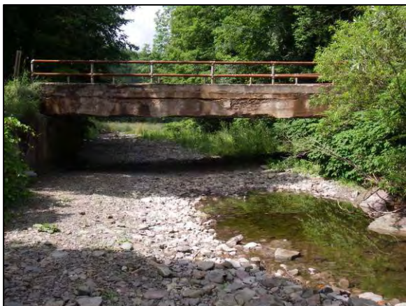
Bridge and Aggradation at Stations 38909 & 39020
