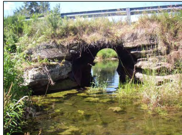
Culvert and Bridge at Station 45598
