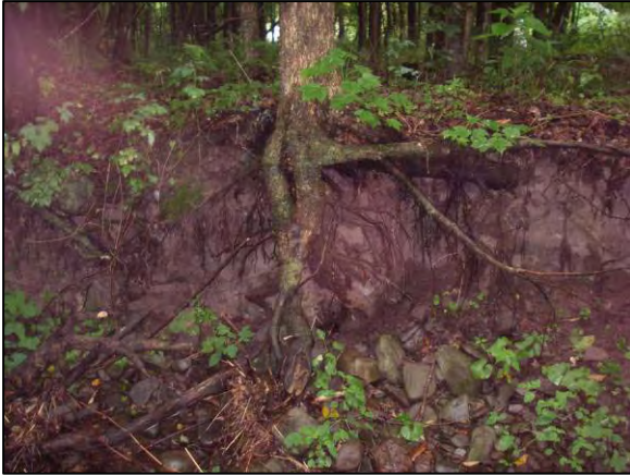
Erosion at Stations 39838 to 39801
