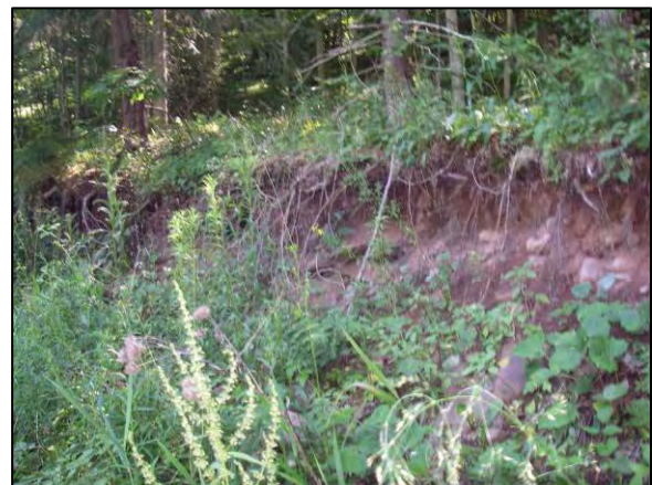
Erosion at Stations 41805 - 41651
