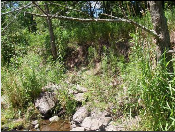
Erosion at Stations 44794 - 44741
