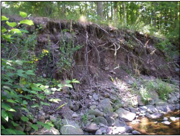
Erosion at Stations 42815 - 42692
