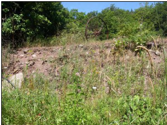
Erosion at Stations 40950 - 40787
