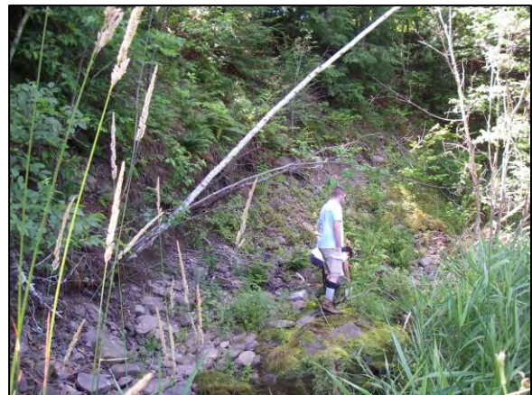
Erosion at Stations 45083 - 44941
