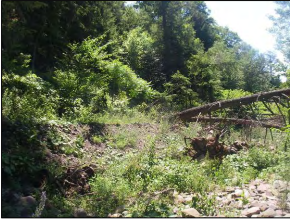
Erosion near Station 39900
