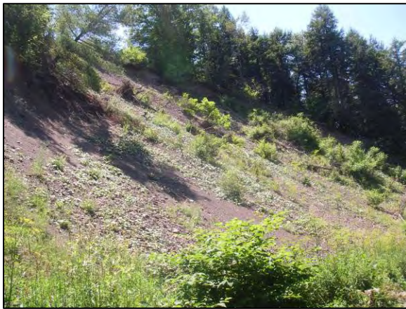
Mass Failure at Stations 40414 - 40265
