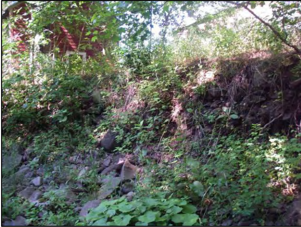
Erosion at Stations 42216 - 42164
