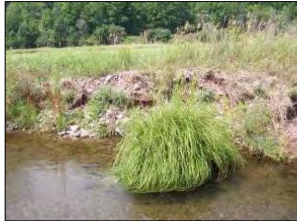
Erosion at Stations 33109 -33010
