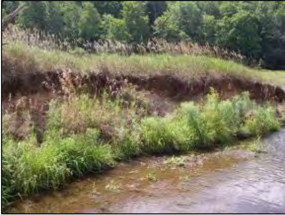
Erosion at Stations 31303 - 31180
