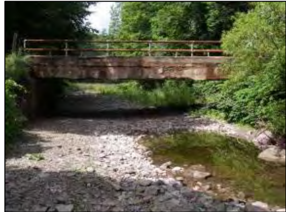
Bridge and Aggradation at Stations 38909 & 39020
