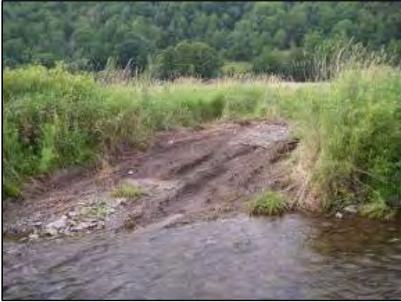
Stream Crossing at Stations 32212
