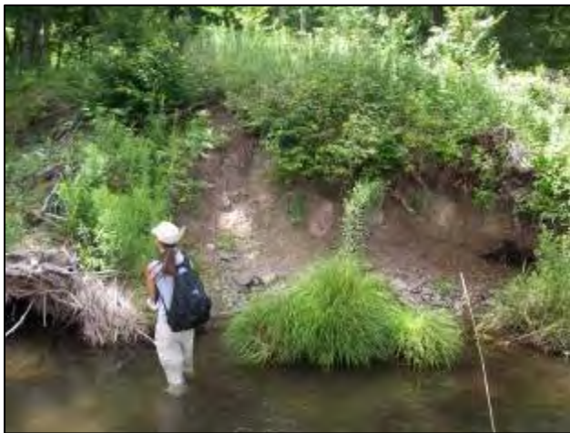
Erosion at Stations 30011 - 29959
