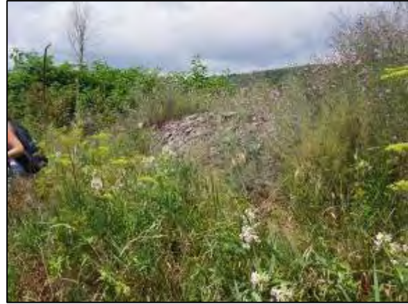
Berm at Stations 37622 -37536
