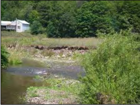
Erosion at Stations 34597 - 34159
