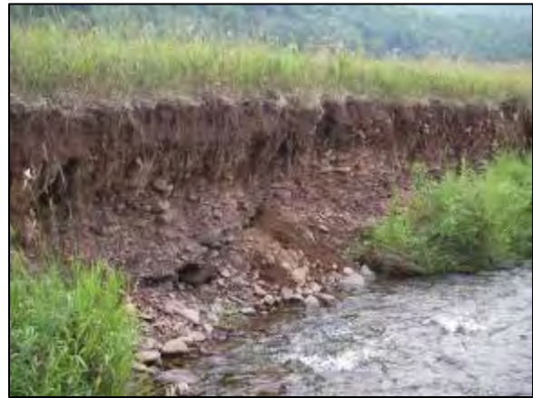
Erosion at Stations 34100 - 33881
