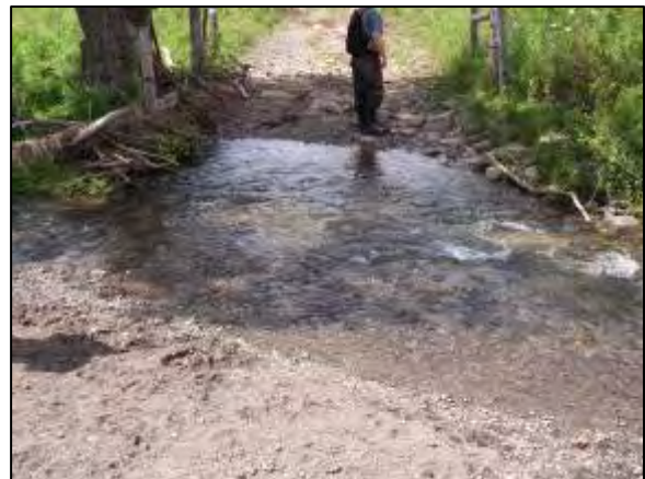
Channel Crossing at Station 28745
