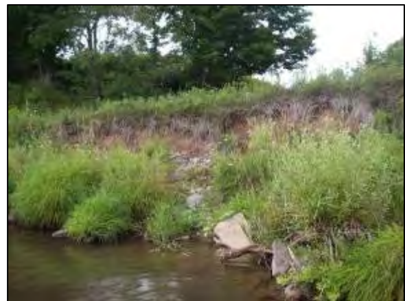
Erosion at Stations 28011 - 27857
