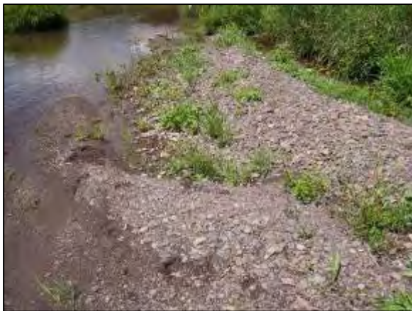
Point Bar at Stations 29549 - 29421
