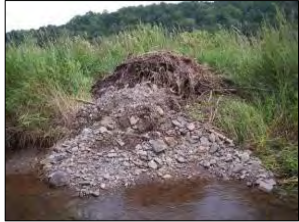
Dredged material from Tributary at Station 32604
