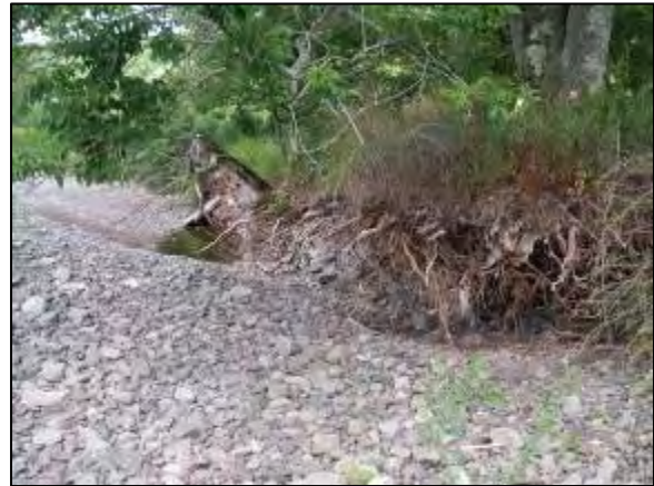
Erosion at Stations 36800 - 36580
