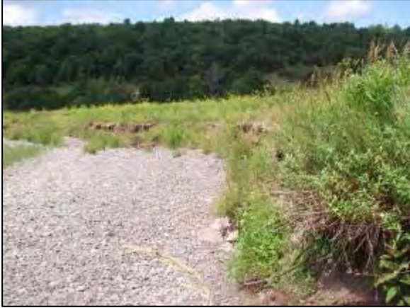
Erosion at Stations 36183 - 34909
