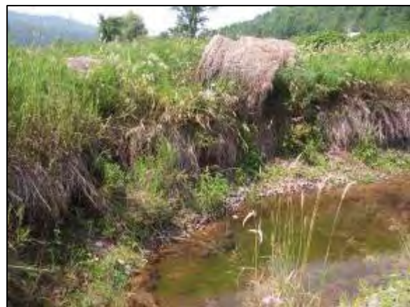
Erosion at Stations 34658 - 34547
