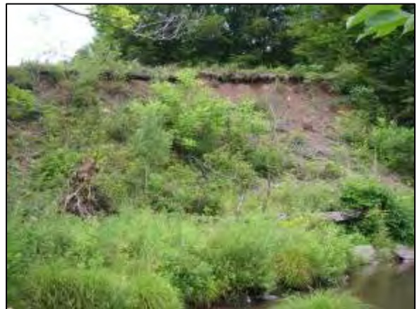
Mass Failure at Stations 27163 - 26938
