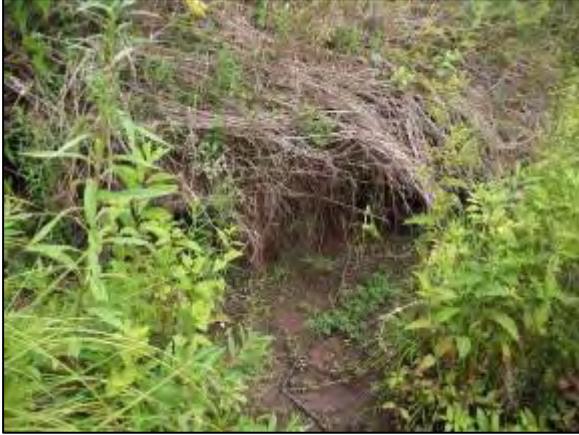
Erosion at Stations 28600 - 28585
