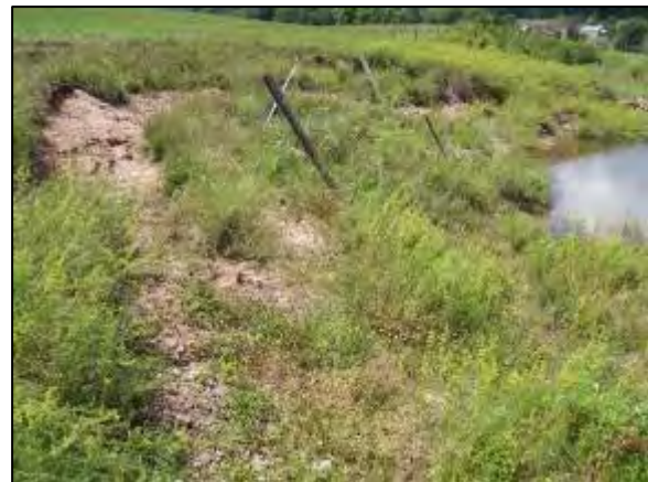
Mass Failure at Stations 29682 - 29664
