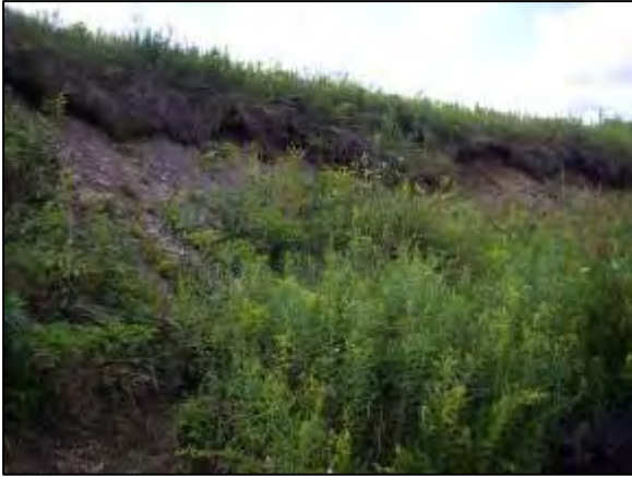
Erosion at Stations 29319 - 29201
