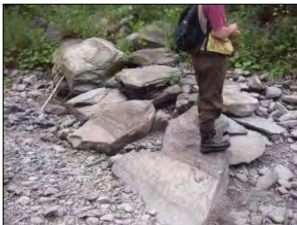
Rock vane at Station 38660
