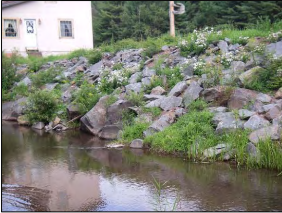
Rip rap at Stations 25485 - 25301
