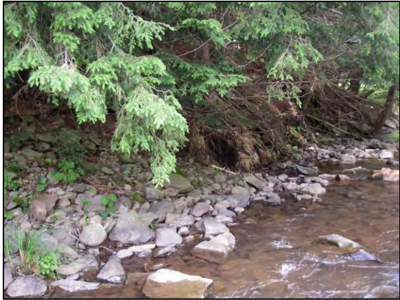
Erosion at Stations 26588 - 26432
