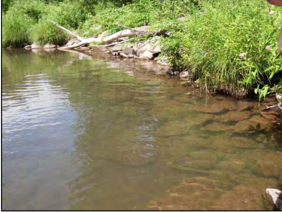
Revetment at Stations 26750 - 26712
