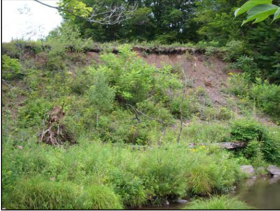
Mass Failure at Stations 27163 - 26938
