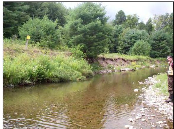
Erosion at Stations 19405 - 19009
