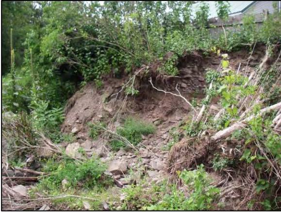
Erosion at Stations 17782 - 17690
