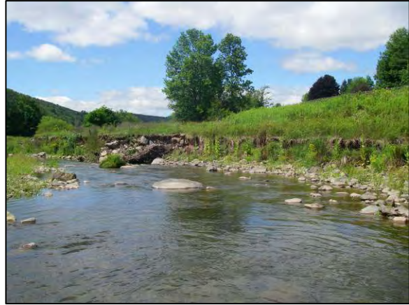
Erosion at Stations 15962 -15500 (downstream portion)
