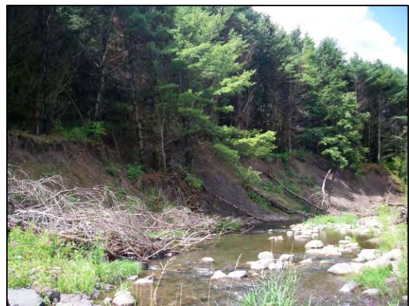
Mass Failure at Stations 16317 - 16052
