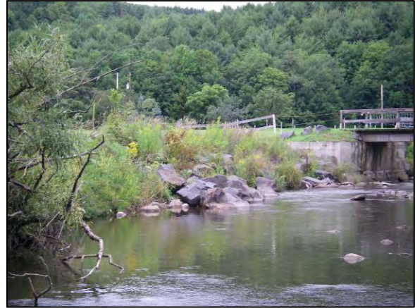
Revetment at Stations 16944 - 16874
