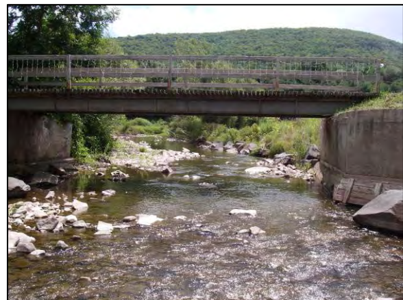
Bridge at Station 16957
