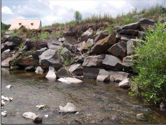
Revetment at Stations 17146 - 16971
