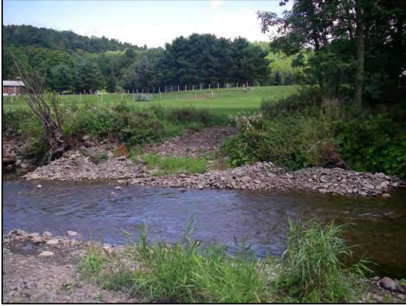
Channel Crossing at Station 15966
