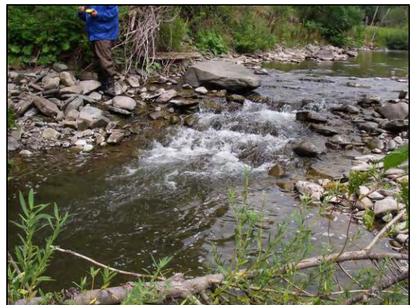
Head Cut at Station 17788
