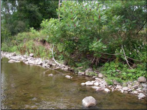
Erosion at Stations 17875 - 17793
