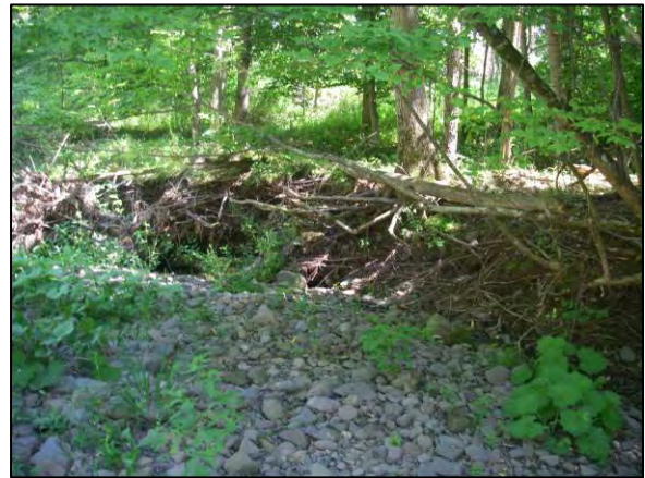
Erosion at Stations 1961-1891
