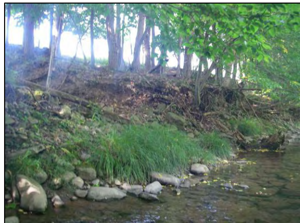
Erosion at Station 4304
