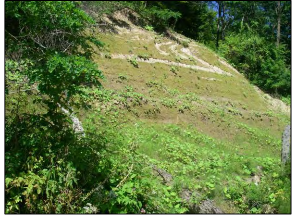
Mass Failure at Stations 2552-2411
