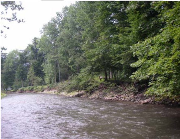
Figure 7 Erosion on right bank, Stns 2300 - 3050
