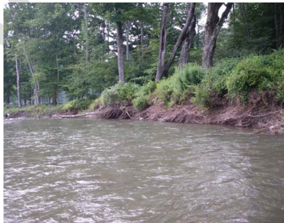
Figure 8 Bank erosion along the baseball field
