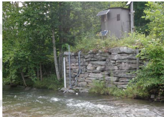
Figure 8 USGS stream gaging station located atop an old bridge abutment on the right bank
