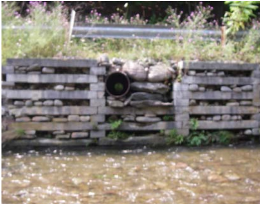
Figure 7 Steel pipe outfall, right bank
