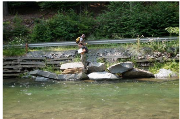
Figure 5 Stn 7700, functional crib wall begins again
