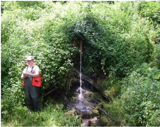
Figure 7 Piped outfall carrying road drainage
