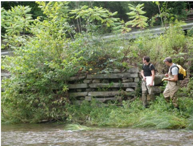
Figure 14 Concrete cribbing revetment, Stn 7870
