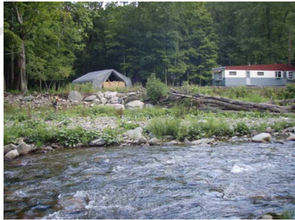
Figure 11 Logs placed to protect eroding bank
