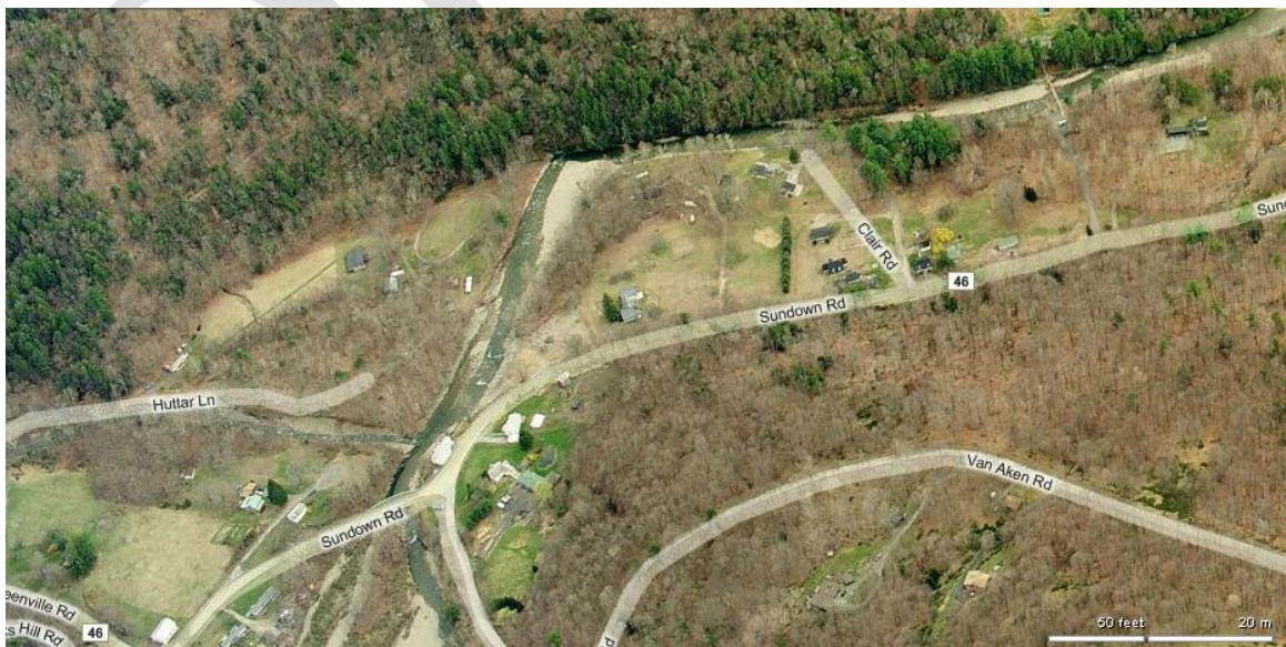
Figure 167 Looking downstream. Complex sediment transport dynamics in MU7
