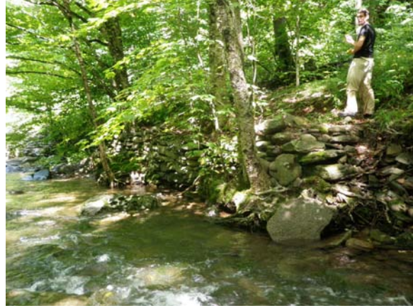
Figure 9 Stacked rock wall, both left and right banks, creating entrenched conditions
