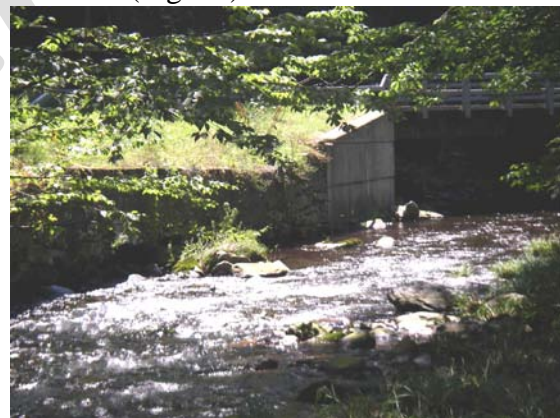
Figure 11 Stacked rock revetment, left bank
