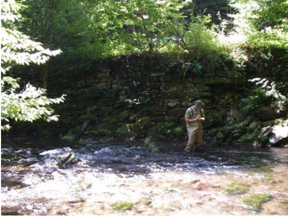
Figure 9 Stacked rock wall, both left and right banks, creating entrenched conditions
