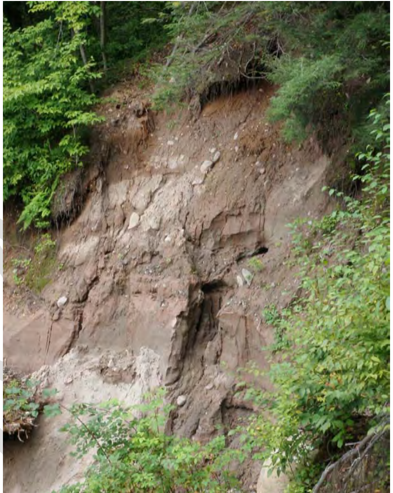
Figure 9 Stratified deposits in high bank, leading to groundwater piping, mass wasting and debris torrent along Greenville Road
