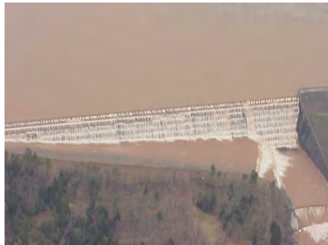
Schoharie reservoir spillway with turbid water following a storm.
