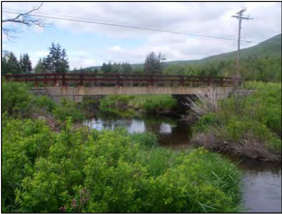
Bridge at Dale Lane
