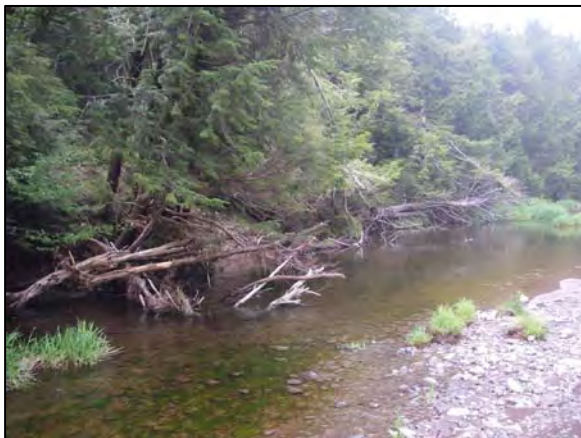
Bank erosion at Station 155250
