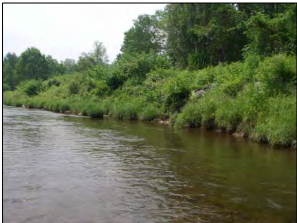
Rip-rap at Station 92040
