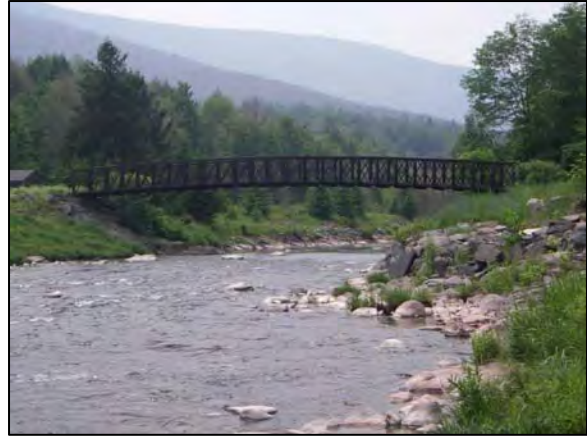
Bridge at Station 91473
