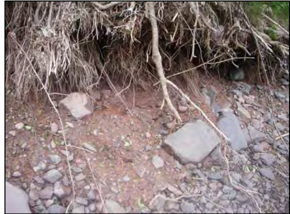
Clay exposure at Station 93150
