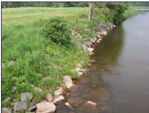
Planting site at Station 97370-95800
