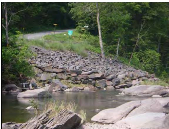
Rip-rap at Station 41200
