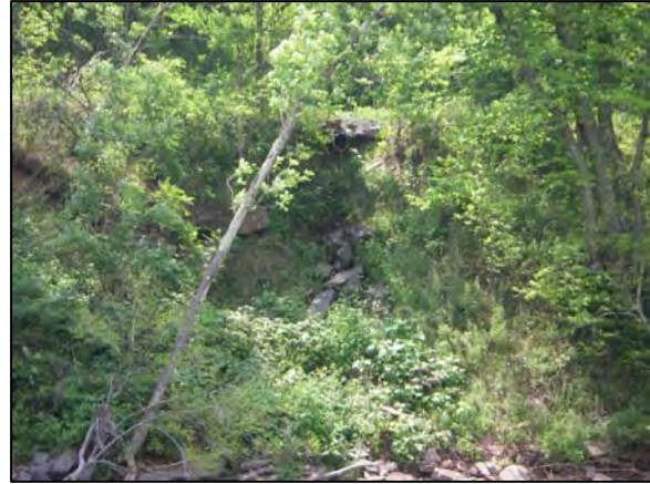
Stormwater outfall at Station 36350
