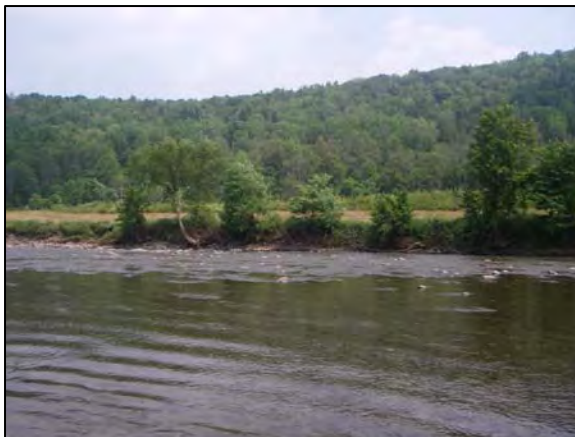
Bank erosion and planting site at Station 40300
