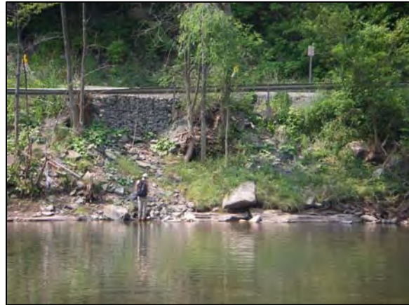
Little West Kill Road embankment
