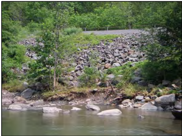
Rip-rap at Station 34050
