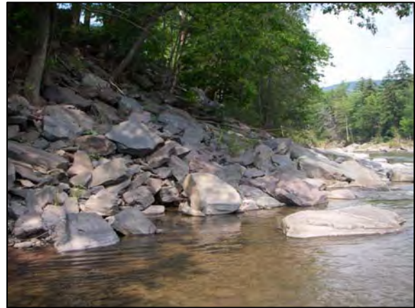
Rip-rap at Station 34360
