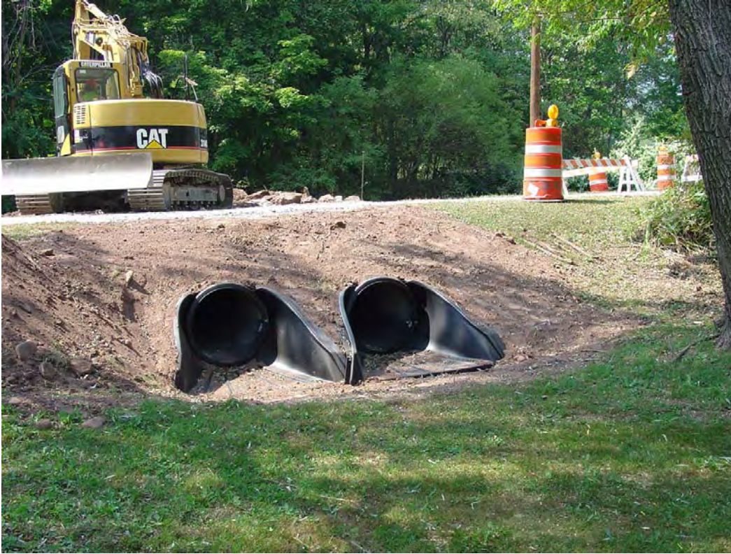
Photo 3: Double 24" CMP floodplain drains installed under road fill.
