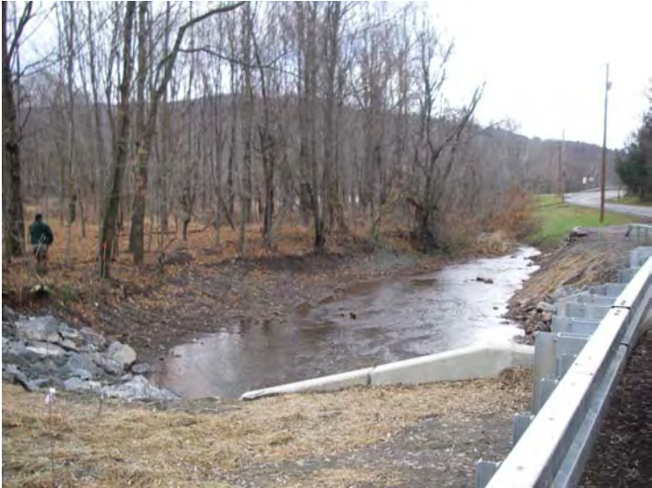
Photo 11: View looking downstream from new culvert
