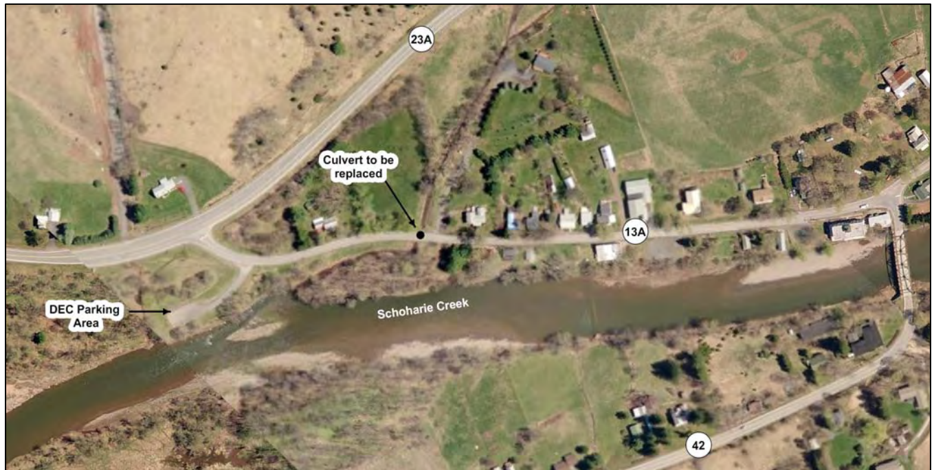
2006 aerial photograph of County Route 13A culvert replacement project site
