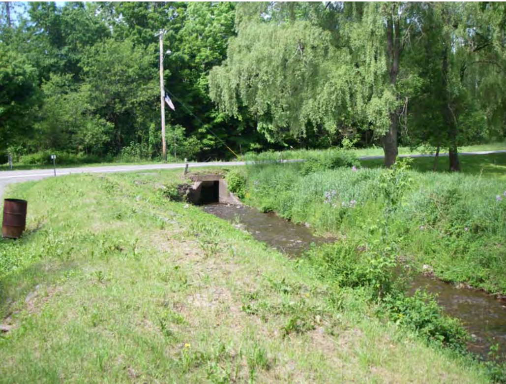
Photo 2: View looking downstream at entrance to existing concrete culvert.
