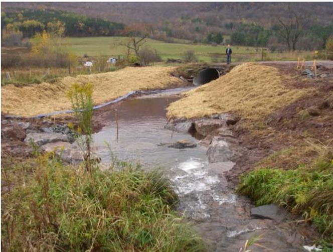
medium rock riprap interplanted with live cuttings of willow and the construction of a cross vane to direct flows and prevent headcutting upstream. The project protects areas planted as a riparian buffer under the CREP.
