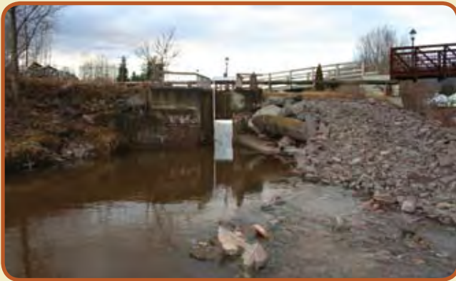
Hunter Mountain takes water directly from Schoharie Creek and diverts it to a vast snowmaking facility with 1,100 snow guns capable of turning water into snow at a rate of 9,000 gallons a minute onto the mountain.
