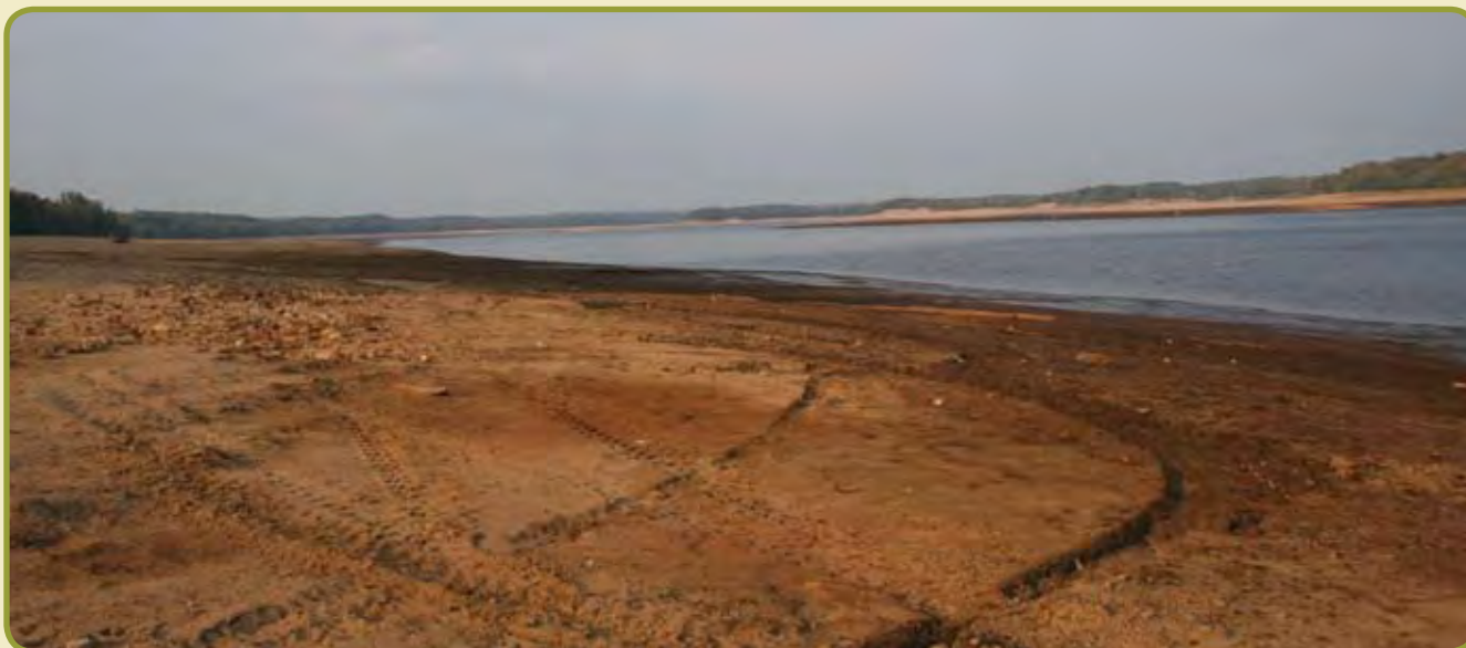
Water levels in Hinckley Reservoir in summer 2007, were 35 feet below the crest and just three feet short of where drinking water supplies would have been affected. The reservoir was only 17% full.
