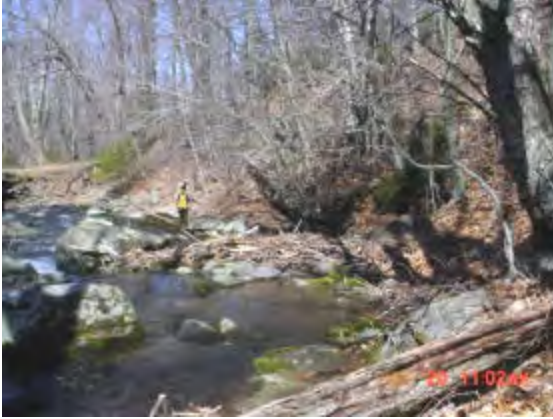
Bank Erosion – embankment, DEC trail at top of bank
