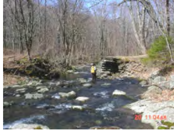
Abandoned bridge abutments, no deck
