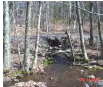
Culverted tributary, looking
