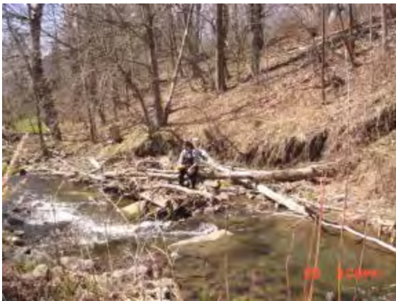
Large woody debris blockage
