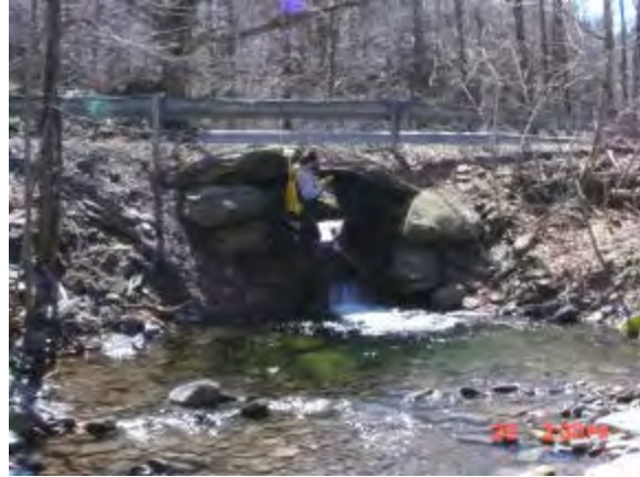
Pettit Brook culvert under Spruceton Rd.
