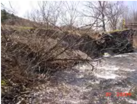
Rip-rap revetment on approach to bridge, left bank
