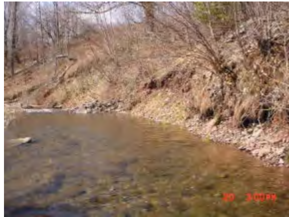
Bank Erosion, with clay exposure, right bank
