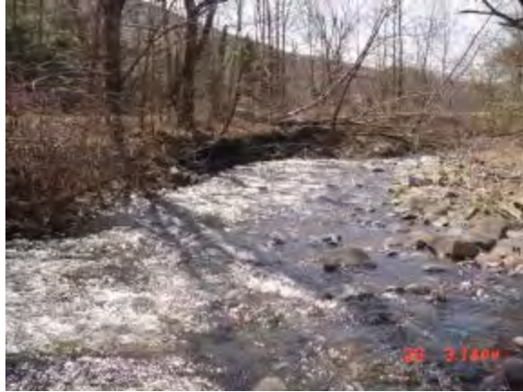
Bank Erosion, left bank
