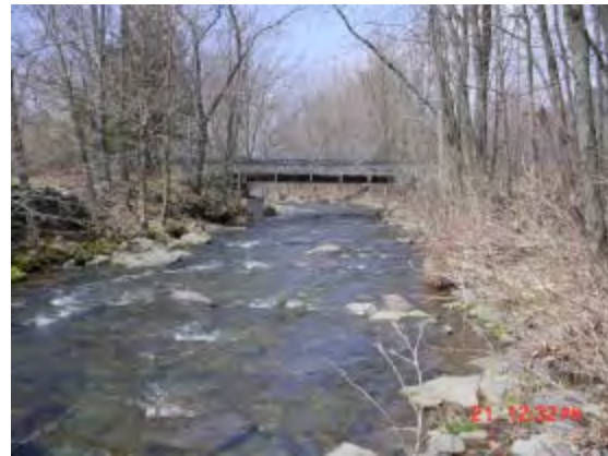
Wolff Road Bridge (TH 147)
