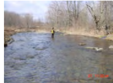
Aggradation - near road embankment, could threaten road in the future
