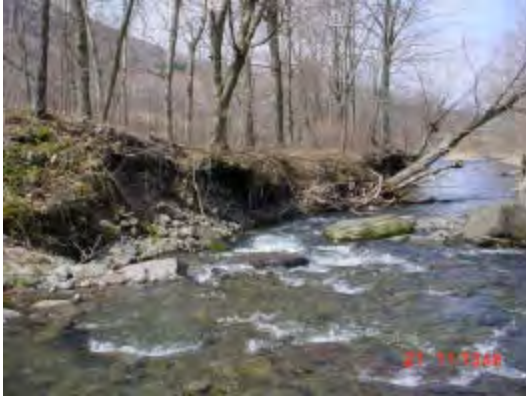
Rip-rap, dumped and stacked at road embankment
