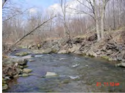
Bank Erosion - some debris introduction, scoured toe and over-hanging vegetation, headcut near up stream end of erosion
