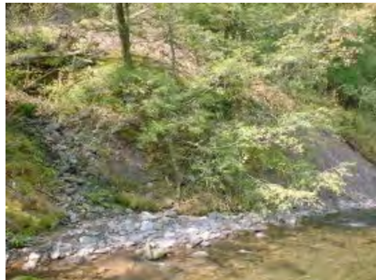
Landslide, with minor toe scour
