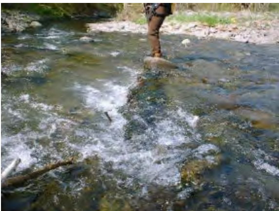
Remnants of habitat structure or crib wall
