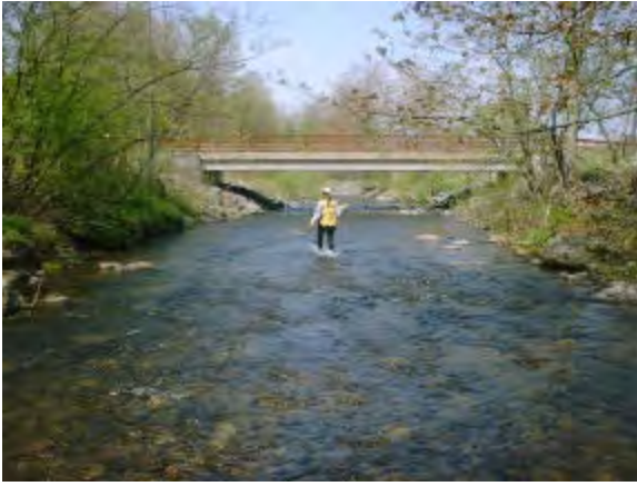
Ad Van Road bridge
