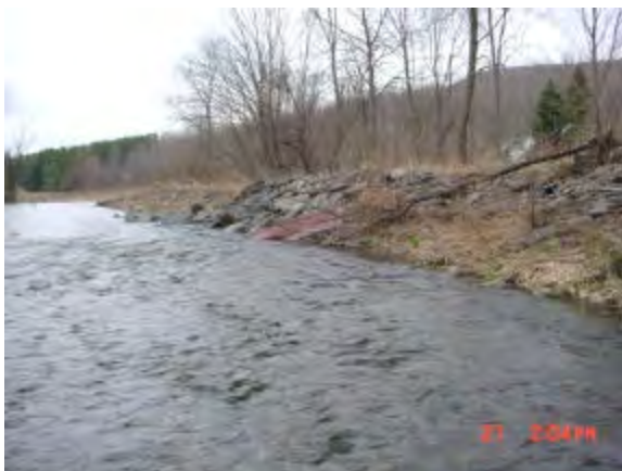
Rip Rap, right bank
