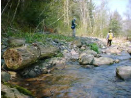
Remnants of log cribbing
