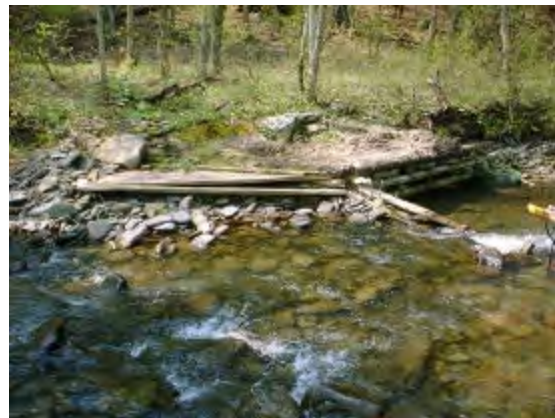
Wing deflector and log sill habitat structure
