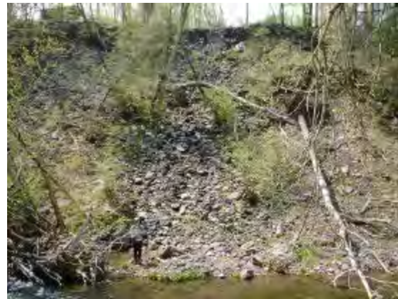
Tributary, Spring on large slope failure
