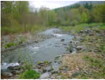
Rip rap, right looking upstream
