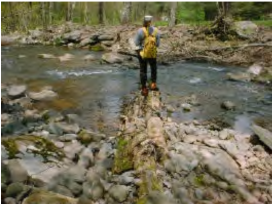
Habitat log sill, breached on right
