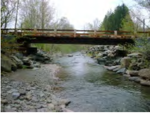
Bridge at Baker Road
