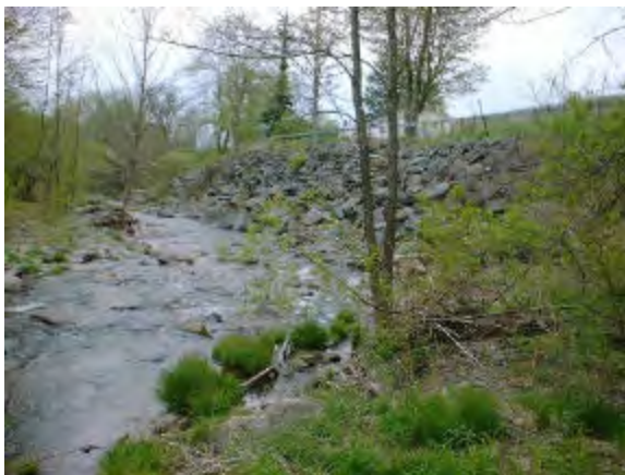
Rip rap, CR6 road embankment
