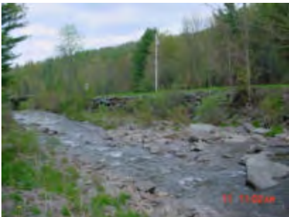
Stacked Rock Wall, right
