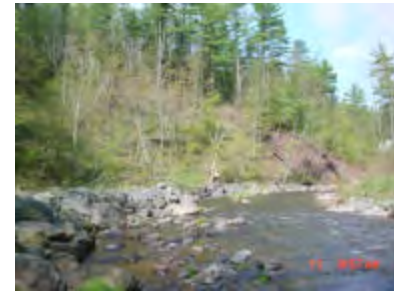
Rip-rap toe protection of slope failure, left bank
