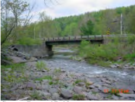
County Route 6 Bridge
