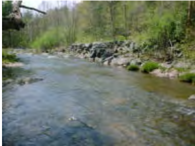
Aggradation adjacent to stacked rock wall
