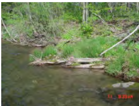
Remnants of habitat structure, right
